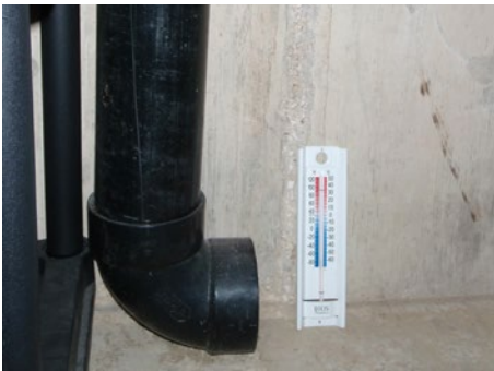
△ Lower vent and thermometer.
